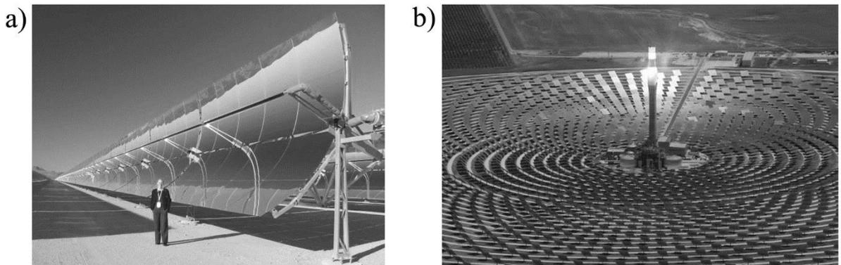
Figure 13 - a) Parabolic Trough Collector, b) Central Receiver System
