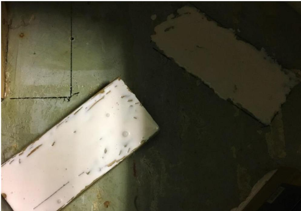
*Figure 45: The underside of a block was covered in glue (left), about to be placed on the fiberglass (right).*
