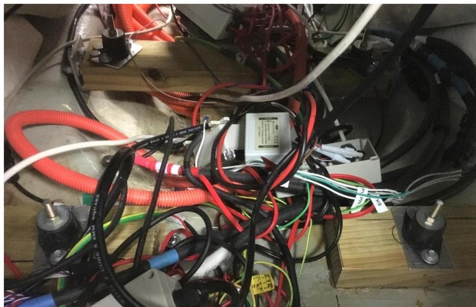
*Figure 49: The Green rubber mounts were installed (corners).*
