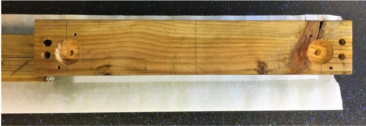
*Figure 44: The wooden blocks and new crossbeam were coated to prevent rot.*
