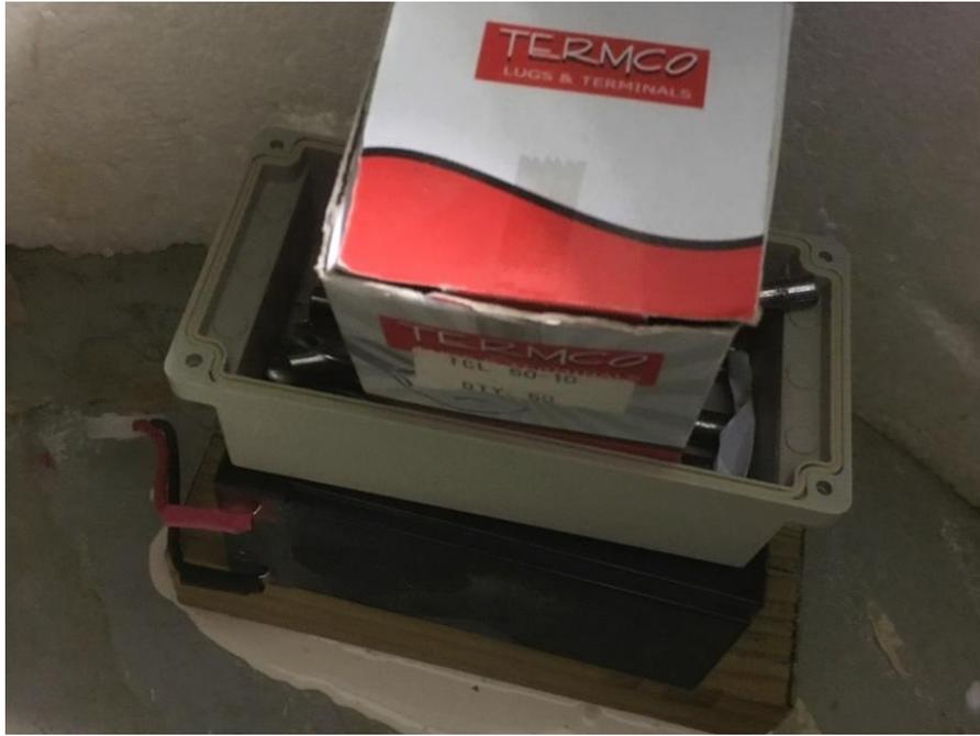
*Figure 46: The block was in place, heavy objects were placed on top to allow for a strong bond to develop while the glue cures.*
