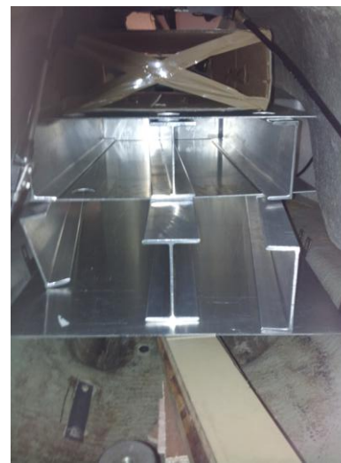
Figure 3.3.7: Battery box test fit
