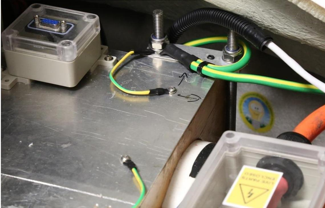
Figure 2 - Auxiliary component mounting plate showing protective earthing conductors.
