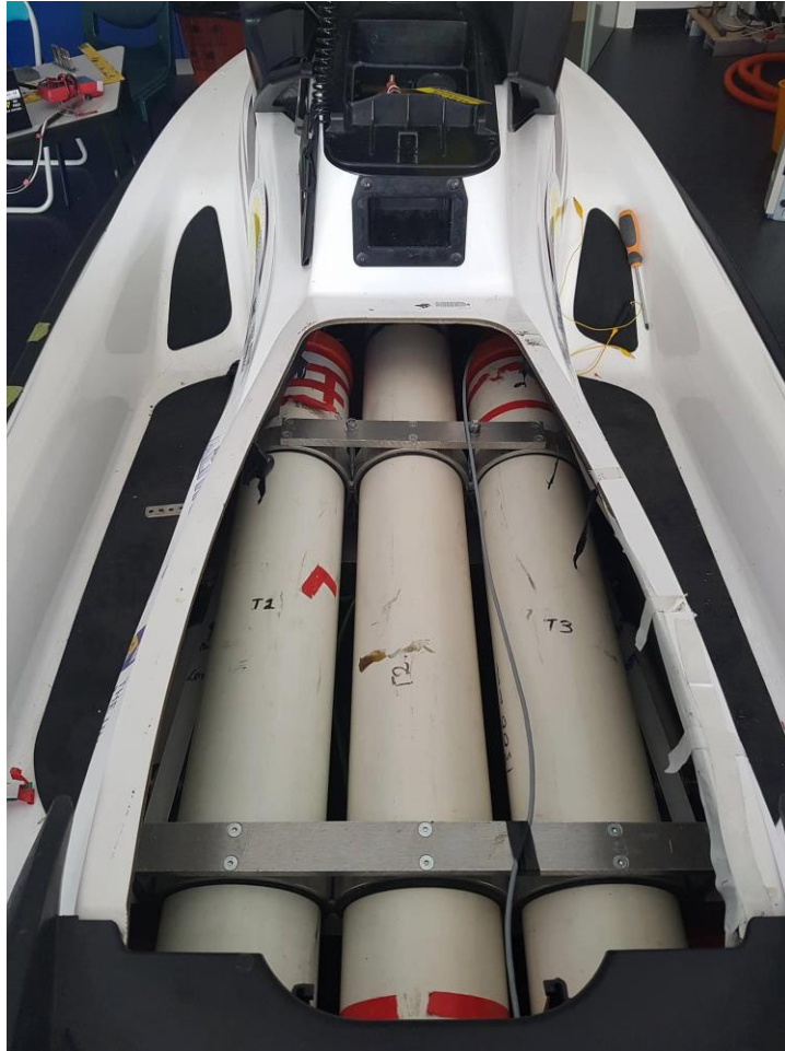
Figure 15: Final battery mount design installed
